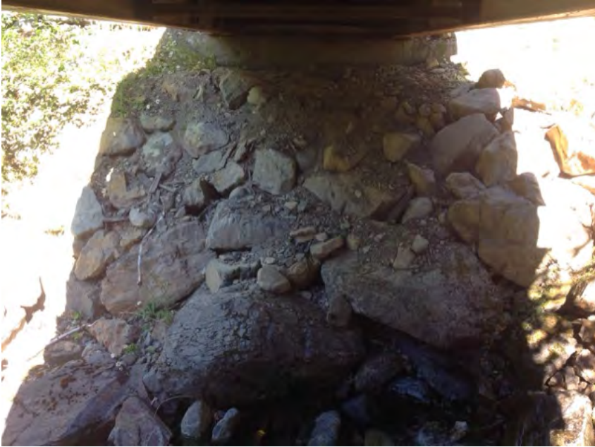
Right Bank Abutment when facing downstream
