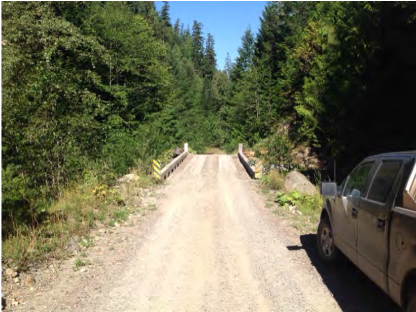
Approach from Left Bank when facing downstream
