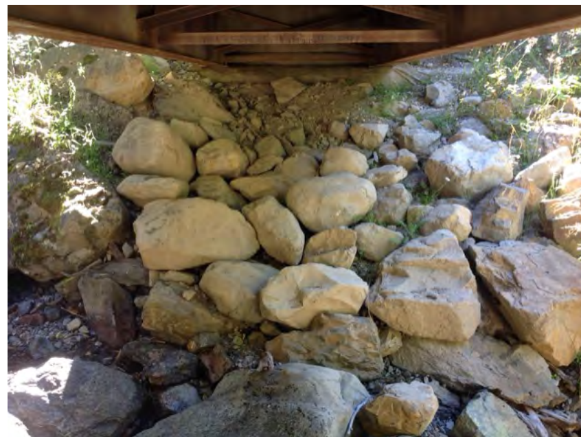
Left Bank Abutment when facing downstream
